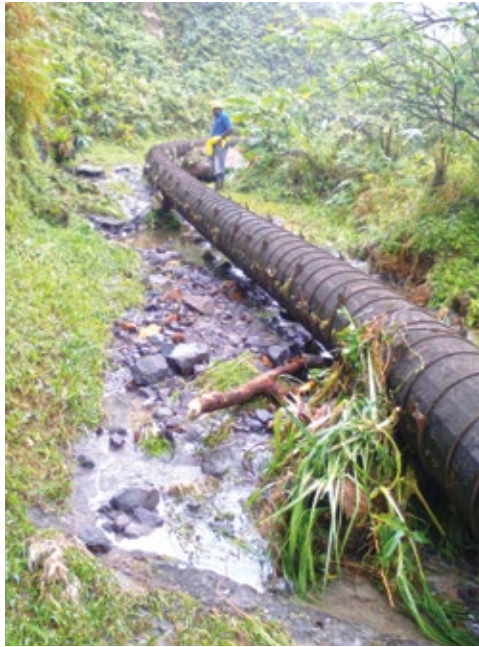
SECTION OF UNDERMINED CLARKE'S RIVER PIPELINE
