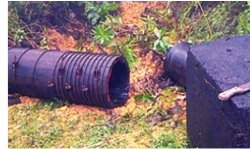
SECTION OF PIPELINE CUT OFF
