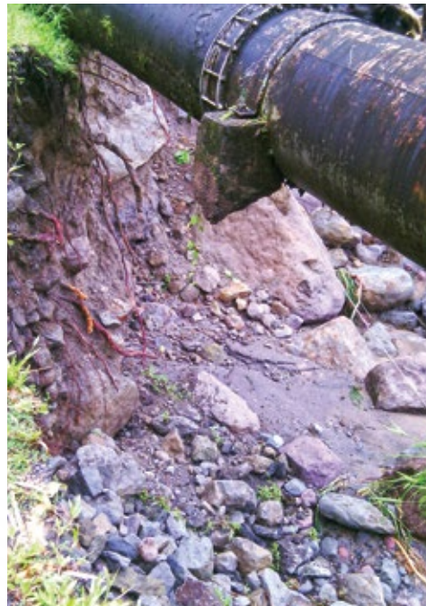
PADU PIPELINE WITH SUPPORT ERODED
