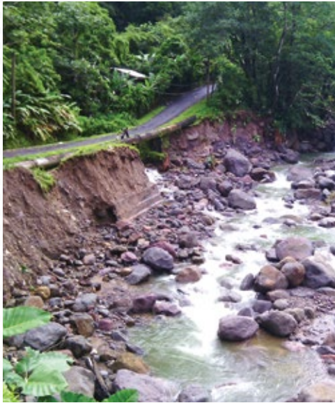
SECTION OF THE UNDERMINED PADU PIPELINE ALONG THE TRAFALGAR PUBLIC ROAD
